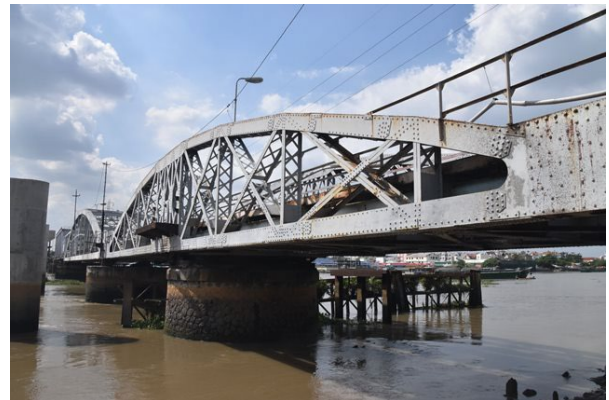
Binh-Loi Bridge, Bien Hoa, Republic of Vietnam { https://saigoneer.com/saigon-heritage/18271-saigon-to-preserve-part-of-old-binh-loi-railway-bridge }
