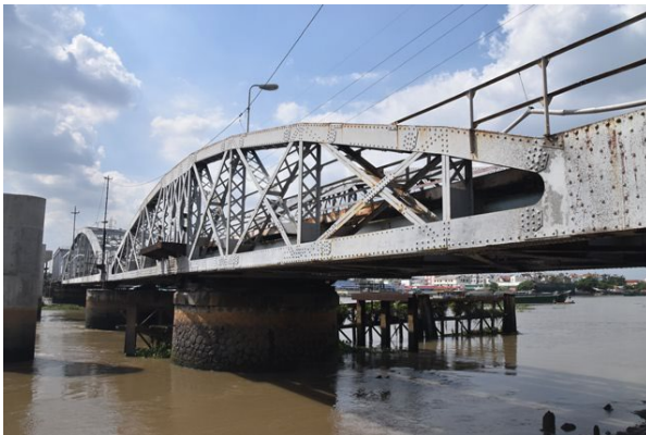
Cầu Bình-Lợi, Biên Hòa, Việt Nam Cộng Hòa { https://saigoneer.com/saigon-heritage/18271-saigon-to-preserve-part-of-old-binh-loi-railway-bridge }
